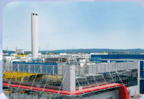
AREVA GBII Facility
