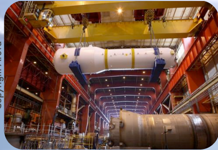
Areva Chalon Plant
